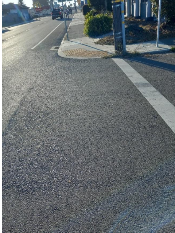
Figure 7: Missing crosswalk markings on T Street at the intersection with 4th Street.
