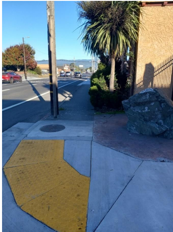
Figure 17: A utility pole and overgrown vegetation partially obstruct a sidewalk on 5th Street.
