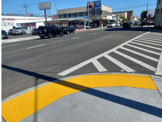
Figure 12: An example of a "blended curb" at 5th Street and Summer Street.
