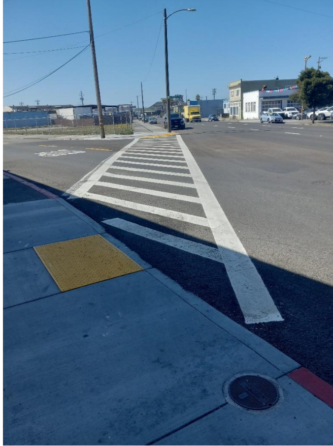
Figure 11: A curb ramp at 5th Street and Summer Street leads into 5th Street instead of into the crosswalk.
