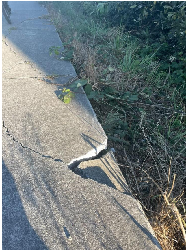
Figure 13: A collapsing sidewalk edge on 5th St near V St on the edge of a steep hillside
