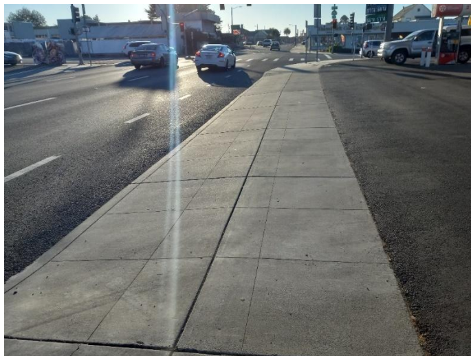
Figure 8: A very long driveway/curb cut at a gas station at 4th Street and R Street/SR-255.
