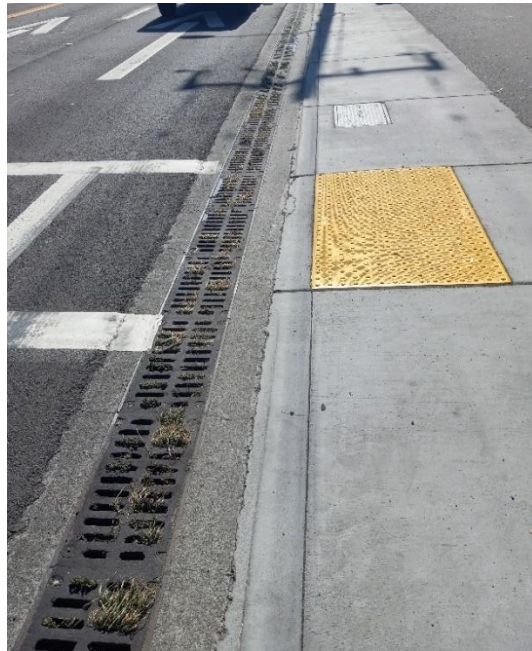
Figure 9: A drainage grate on Broadway identified as a hazard for cane users.
