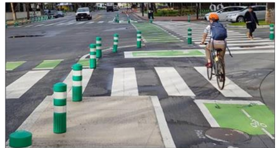
CALBIKE: QUICKBUILD BOLLARDS
