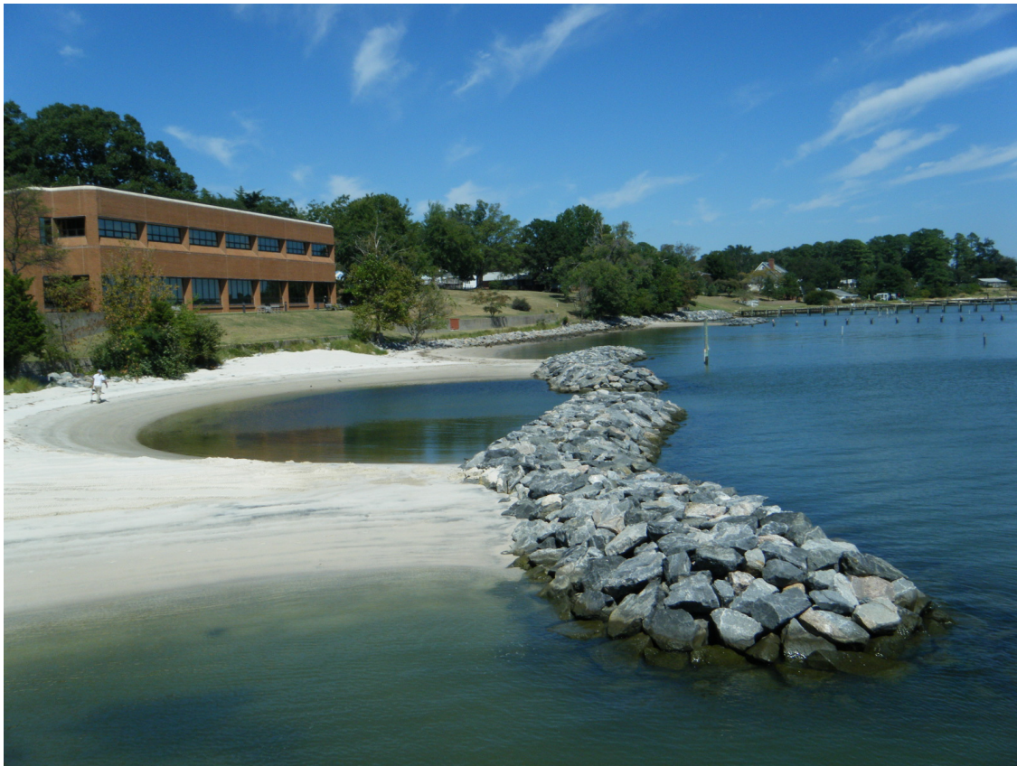
Figure 8: Breakwater system. Source: Virginia Institute of Marine Science (2017)
